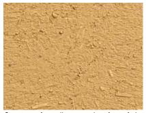
Structure of a well-prepared surface of clay undercoat plaster
