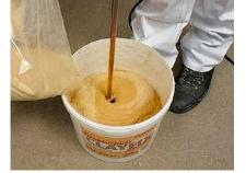
Mix the content of the bucket into water. Then leave to soak for 30 minutes.
