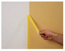
Removing after wiping over
