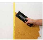
Applying the first colour up to the masking tape
