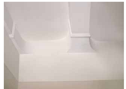
Ceiling with plaster-clad beams, rounded valleys and stucco mouldings
